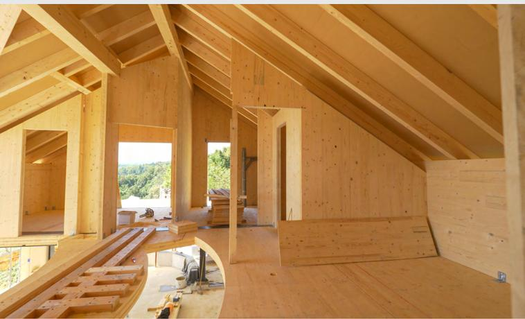
CLT (Cross Laminated Timber) construction is an innovative method that uses structurally reinforced timber panels, creating sustainable and modern buildings.
